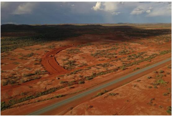
Figure 2: Commencement of Construction of Haul Road at Intersection to Public Nanutarra Road (foreground) (March 2022)
