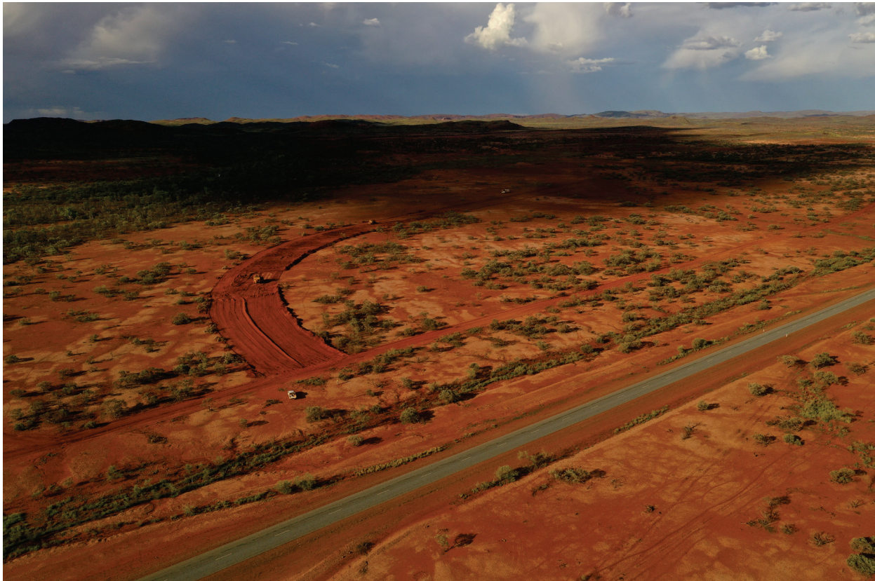
Figure 2: Commencement of Construction of Haul Road at Intersection to Public Nanutarra Road (foreground)
