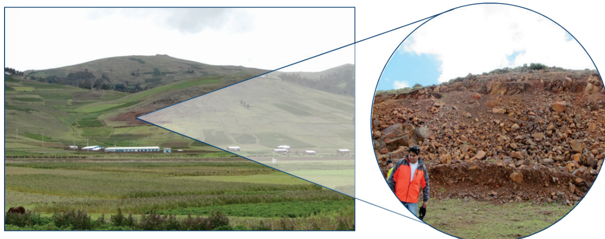
Figure 7: Opaban 1 deposit has favourable topography for low strip-ratio, open cut mining
